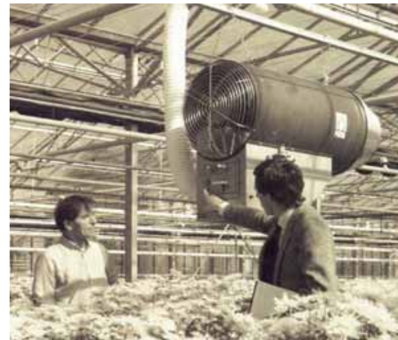
Verwarming + CO 2 generator in chrysantenteelt (1984).
