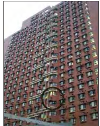
Two rooms located in adjacent upper and lower floors in a student dormitory were selected for tracer gas measurements.
