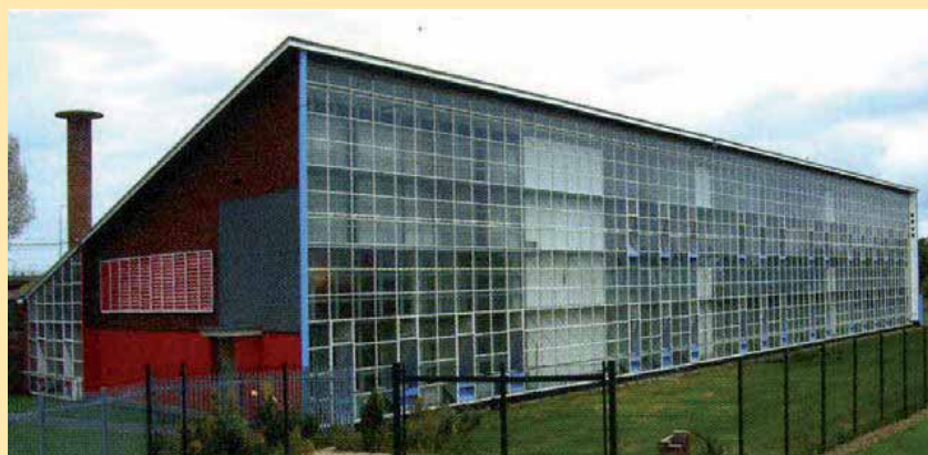
St. George's County Secondary School in Wallasey in Cheshire, England. Foto: Jeremy Marshall [9].
